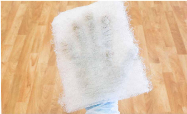
Adhesive based sheets are used on the first pass of the floor.
